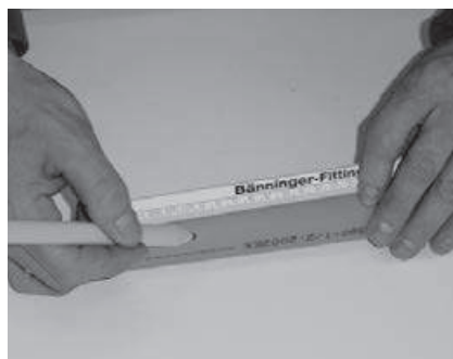
Fig. 5 Mark out the socket depth.
