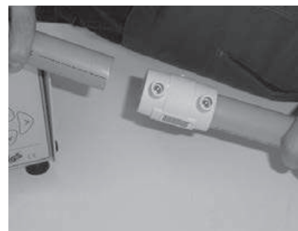
Fig. 6 Push in the socket up to the marked position on the pipe.
